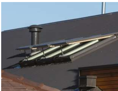
Pitched Roof Skylights
