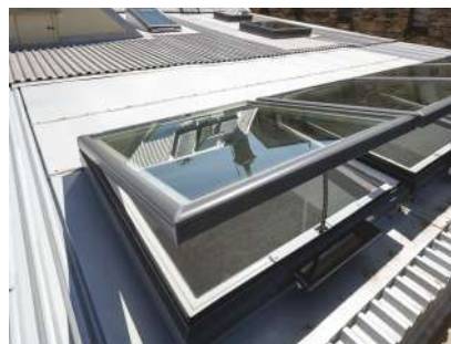
Flat Roof Skylights
