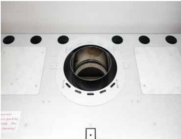
2. 6" Flue fitted. Note: crimped end is down. Must connect active pipe using stainless steel rivets or self drilling screws. 2 for each joint.
