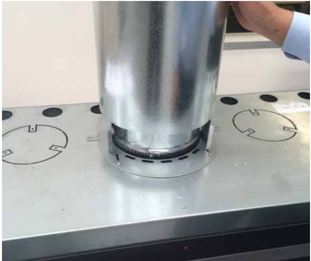
5. Air cooled bracket and pipe fitted to unit. The outer casing of the flue (10") must be raised 75mm above the zero clearance box.
