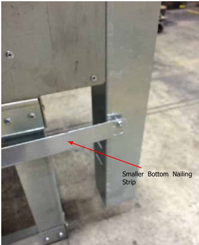
Nailing strip installed with slotted side on unit. The slot allows the movement of the nailing strip to be adjusted depending upon thickness of finish material.
