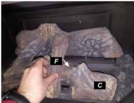
Log F install
