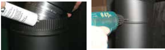
Secure 90° elbow to vertical pipe with Mill-pac and 3 screws.
