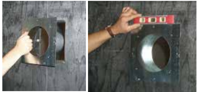
Wall Thimble - level & secure with 4 screws.
