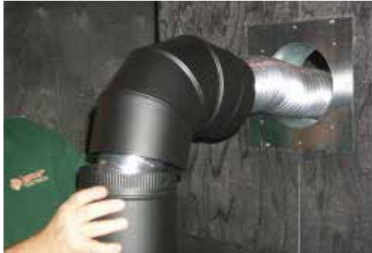
Slide 90° elbow over flex
