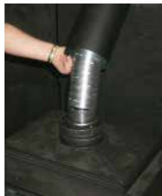
Fit flex over adaptor and secure with Mill-Pac and 3 screws.
