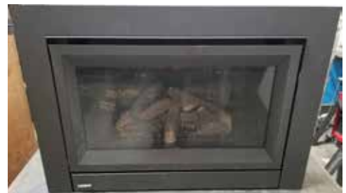
Completed Faceplate & Safety Screen Installation
