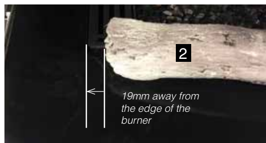
Log 2 in position
